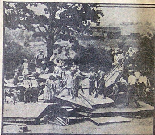
Any wind that blows down a school house is all right, according to the children shown in this picture playing in the ruins of a portable school at Bairdford, near Pittsburgh, Pa. A sudden gale blew the building a hundred feet from its site and effectually flattened it.
